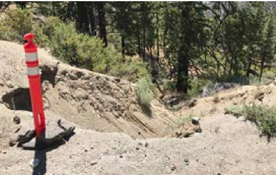
10 Significant erosion of the roadway corridor from winter storm runoff.
