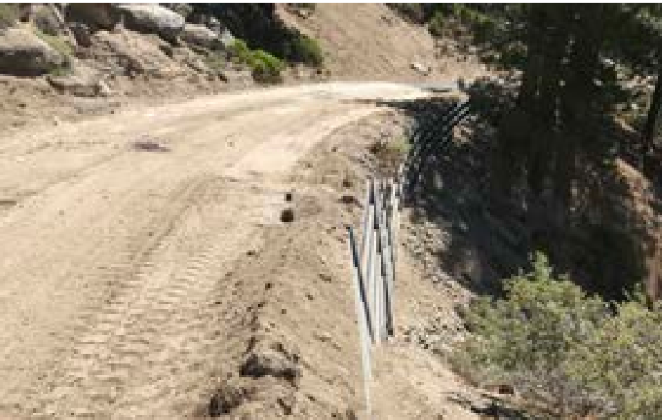
4 Area where the roadway corridor has been reinforced with an engineered retaining wall.
