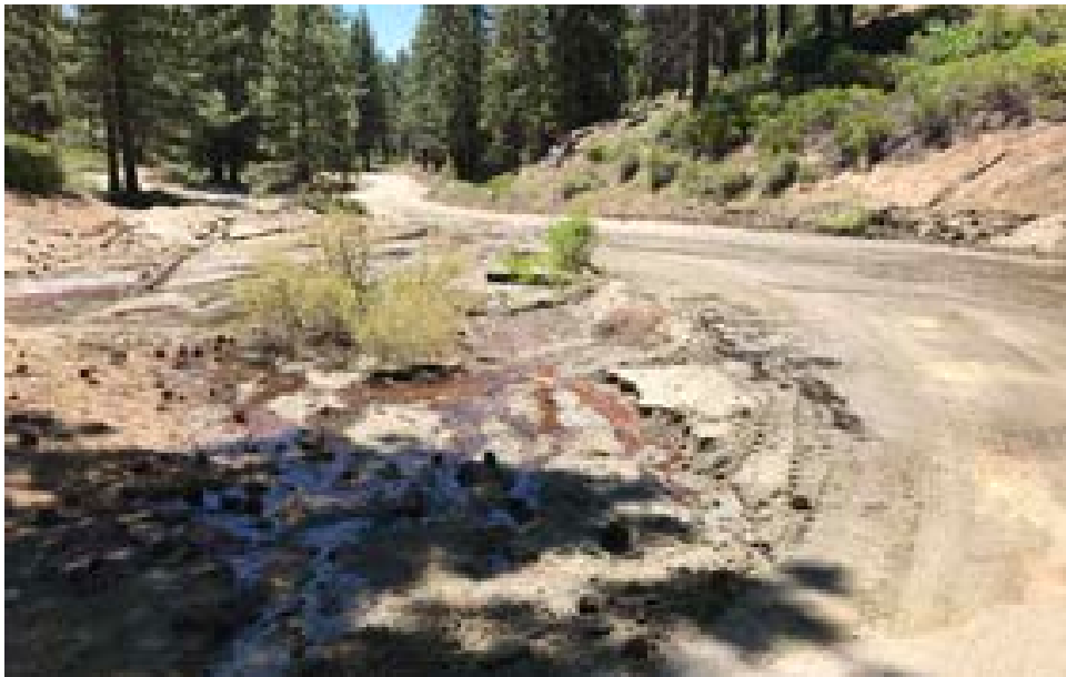
13 Runoff from the adjacent hillsides moves across the Kingsbury Grade corridor, eroding the road surface.
