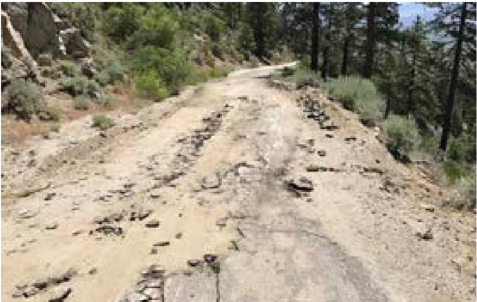
17 Degraded asphalt roadway from insufficient drainage and maintenance.
