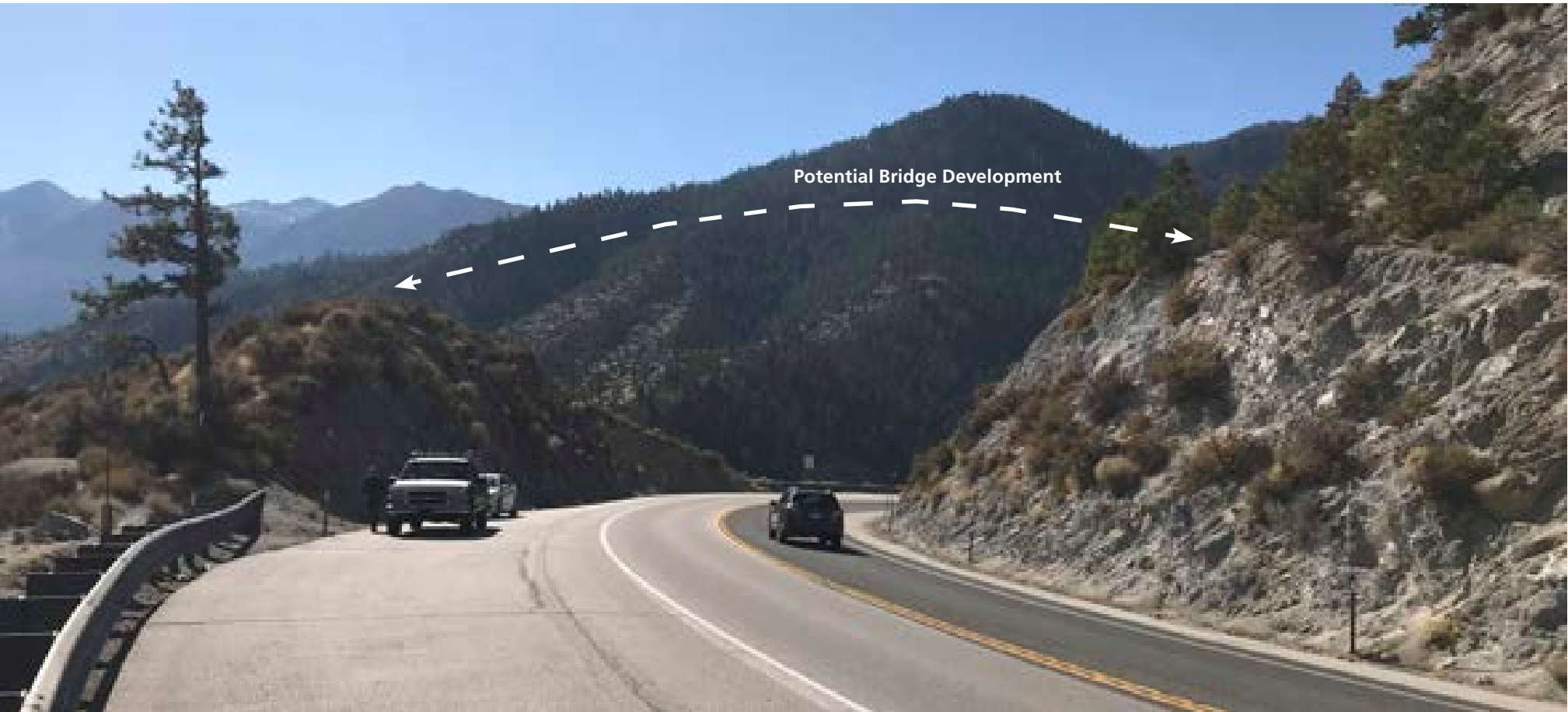
Location where SR 207 has been cut into the hillside, leaving elevated slopes on both sides of the roadway corridor
