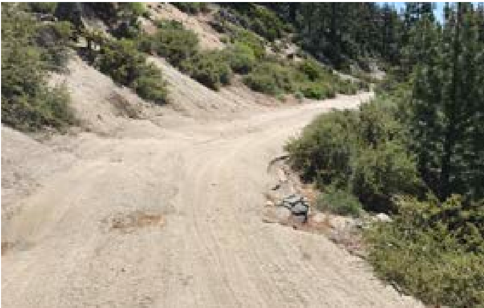
6 Typical impacts from erosion where drainage off of the hillside degrades the asphalt surface over time.
