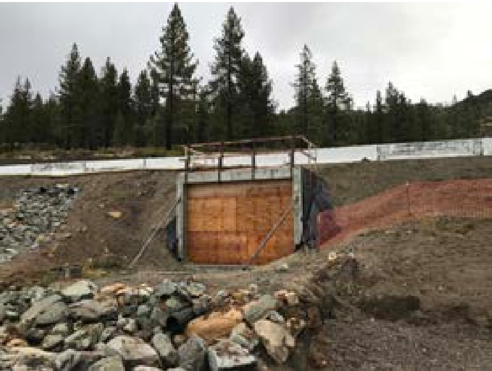
Tunnel underpass being constructed for the Stateline to Stateline Bikeway trail
