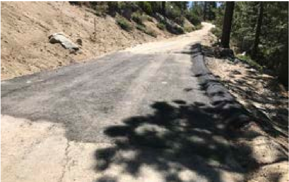
5 Newly surfaced asphalt treatment where winter storm erosion washed away the roadway corridor.
