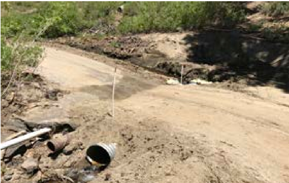
15 Severe trail tread erosion where multiple culverts have been placed to facilitate drainage.
