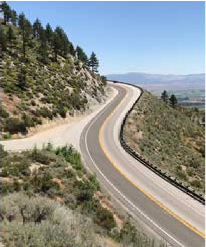
Blind turns and a narrow right-of-way at the lower SR 207 junction requires costly design interventions to cross
