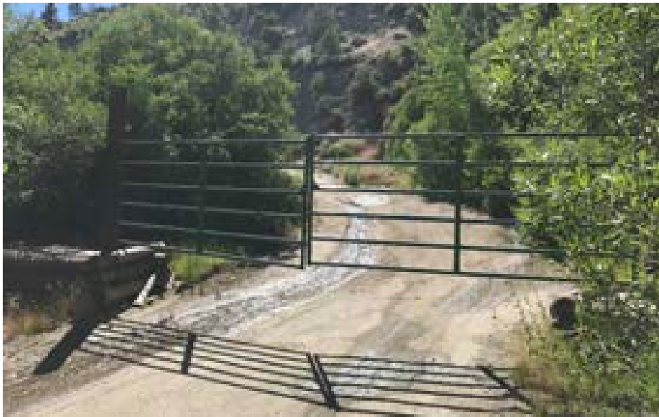
2 Entry gate at the lower crossing point with runoff from the adjacent hillside eroding the existing trail tread.
